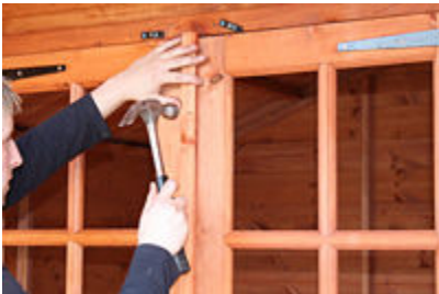
30.Photo Fix the door cover strip. Nail using eight 25mm nails onto the door with the handle
