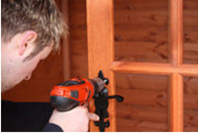
29.Photo Fasten the handles to the door using 25mmx8g screws. The handles must operate freely.
