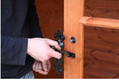
28.Photo Assemble the door handle.
