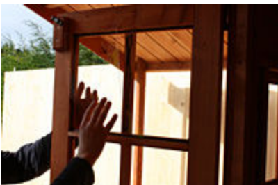
34.Photo Place the pane in position and press onto the silicone making sure the pane has sealed all the way round. Some panes may require easing using a medium sand paper to sand down the edges.
